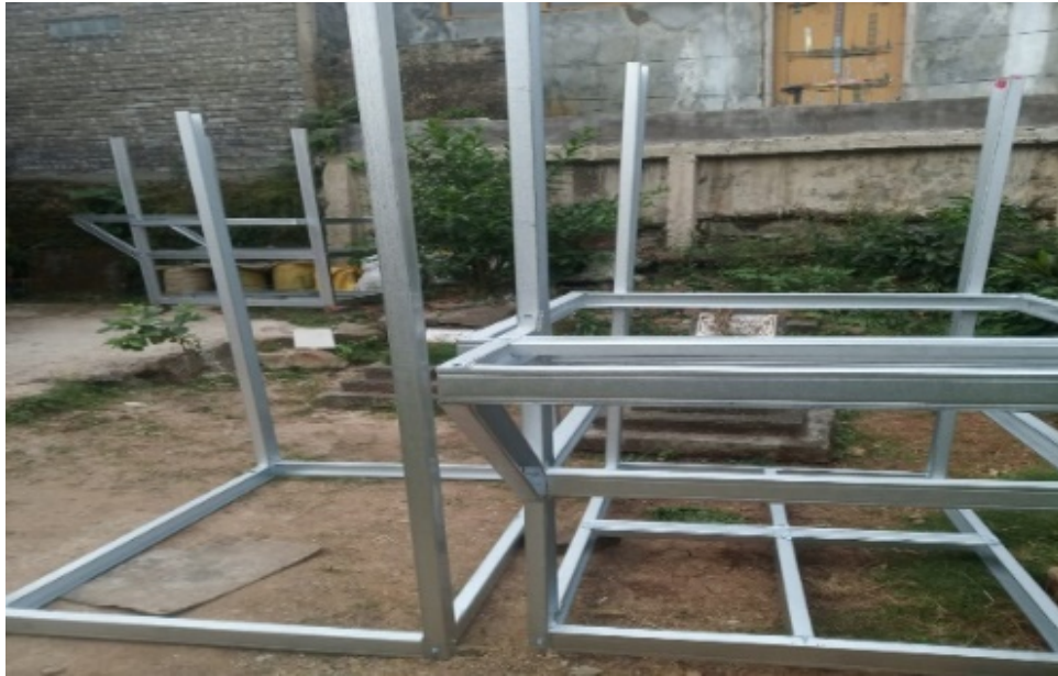
Fig. 6. Assembly of aquaponic pond supports
