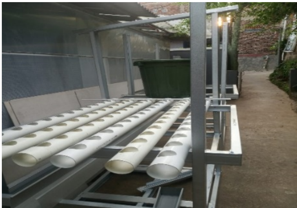
Fig. 7. The installed aquaponic system
