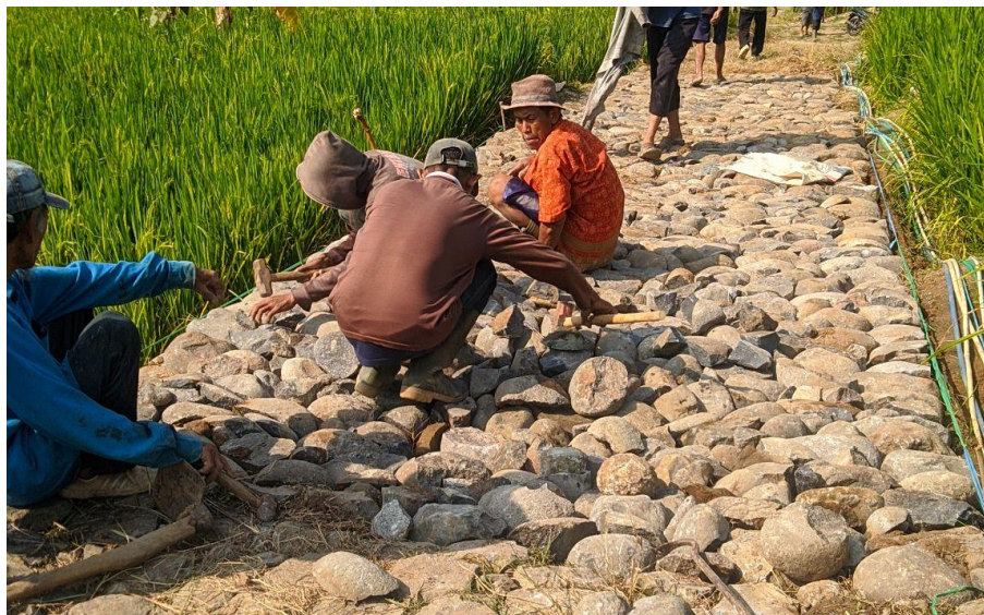
Fig. 1. Residents carry out road repairs to facilitate the mobilization of farmers
