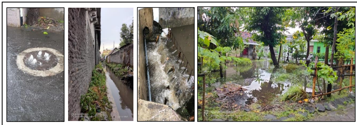
Fig. 4. Picture of Drainage Overflowing to the Road and Puddles in Slum areas
