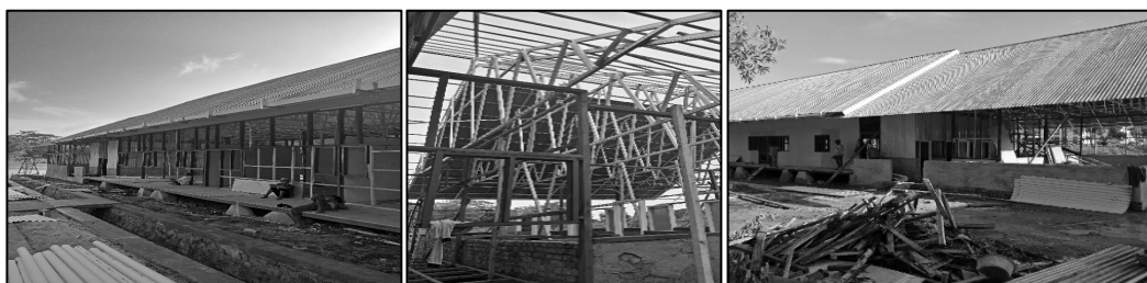
Fig. 6. Employee lodging construction progress
